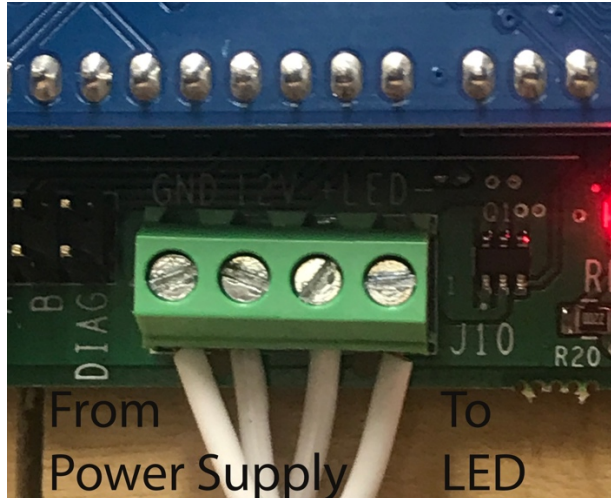
Figure 2: LED Wire Installation
